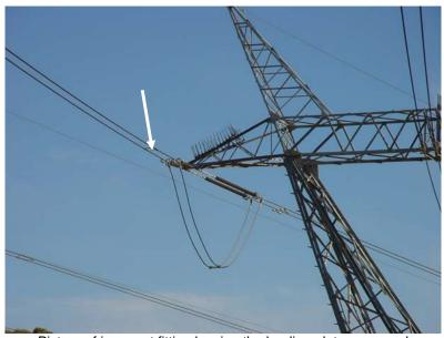
Picture of incorrect fitting leaving the landing plates exposed
